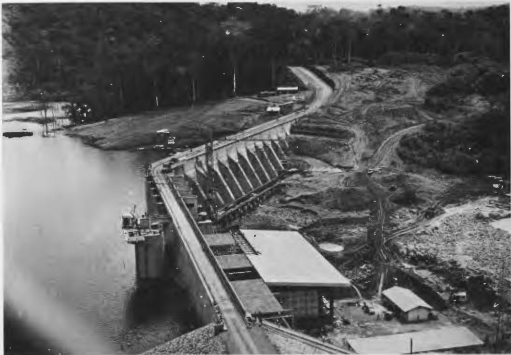
Figure 13.--Hydroelectric dam at Ayame on the Bia River. This dam has a capacity of 80 million KWH per year. Most of the current is used in Abidjan. Courtesy of Republique de Cote d'Ivoire, Direction de l'Information.
